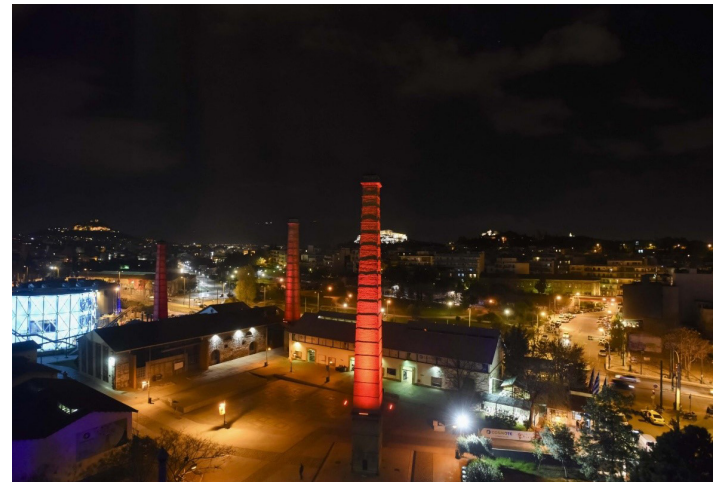
Current view of the plant's central courtyard with its illuminated chimneys. (source, studio kominis, https://gasmuseum.gr/en/history-and-collection/ )
