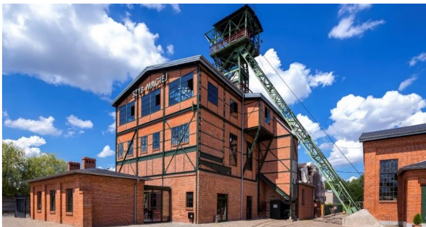
Figure 12 Maciej Shaft, Zabrze ( URL8 )
