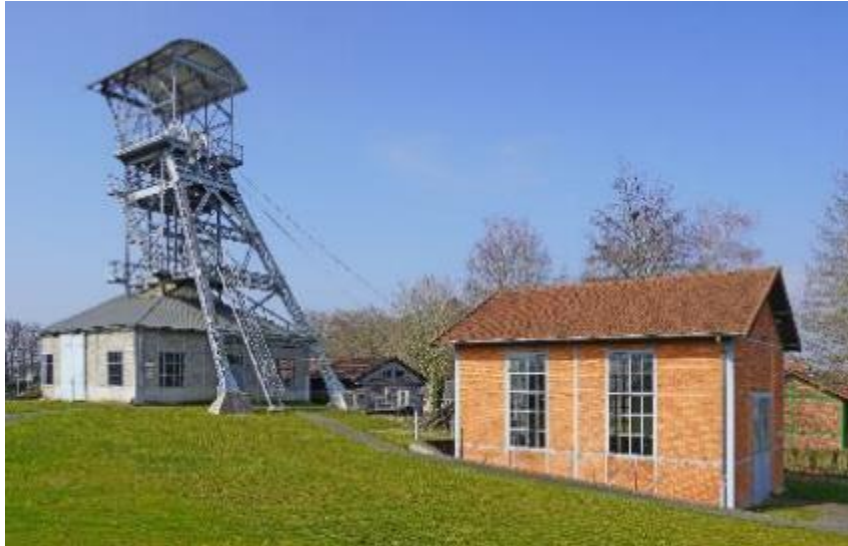
Figure 100. . The Glénons shaft, complete with headframe, electric extraction machine and fan [14].
