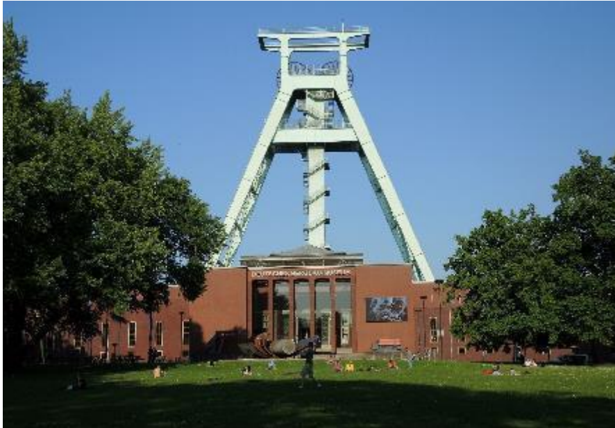
Figure 41. Front view of the German Mining Museum in Bochum [© Von Christian Nawrot].
