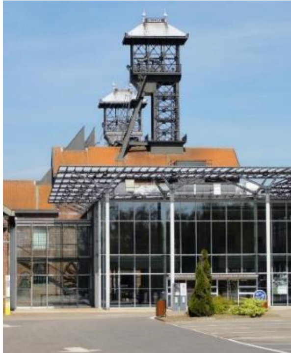
Figure 92. The entrance of the Mining Center [9].
