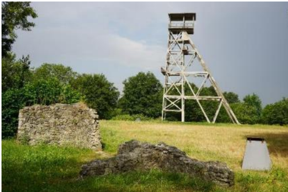
Figure 95. The Epagne headframe is made of concrete [10].
