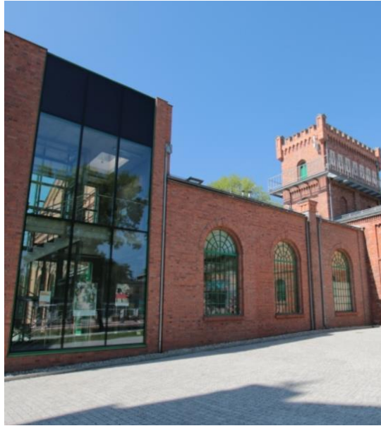
Figure 8. Saturn Mine and GSW Power Plant [135].
