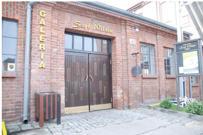
Figure 11. Wilson Shaft in Katowice [15].
