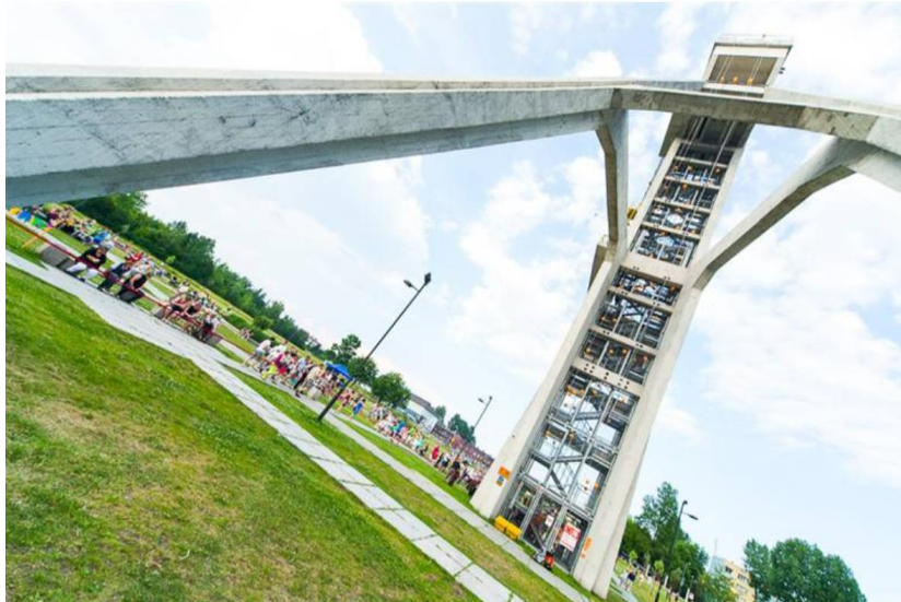
Figure 17. President shaft in Chorzów - Szygarka Complex [140].
