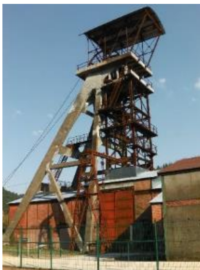
Figure 98. Headframe of the Puits Ricard mine in La Grand'Combe (Gard department) [1].
