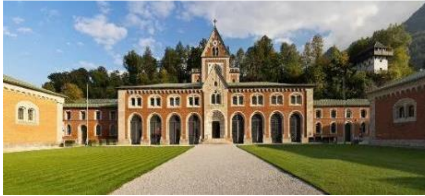
Figure 52. Old salt works main facility at Bad Reichenhall [© Jörg Braukmann].
