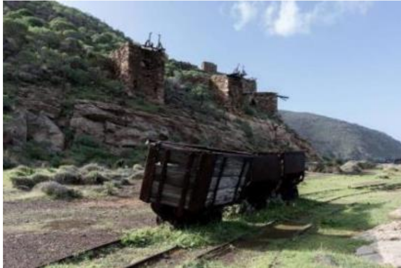
Figure 71. The mining area of Mega Livadi, the core of the study of the Serifos open-air museum [47].
