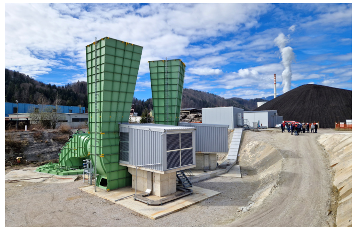
Figure 16. New Preloge II Ventilation Shaft (photo: PV archive).
